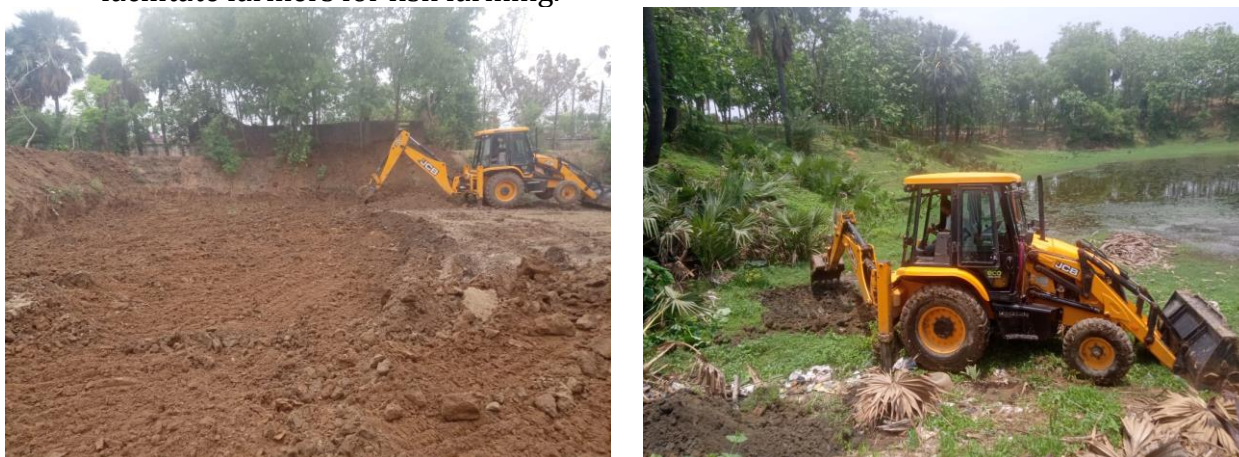
Fig: Desilting of Pond
