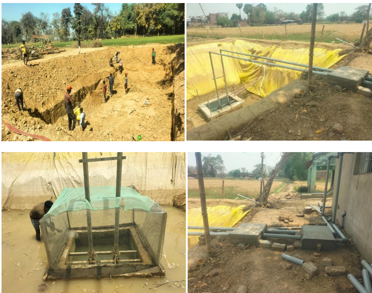
Pic: Construction of Water Tank and piping system linking to filters under Pump house
